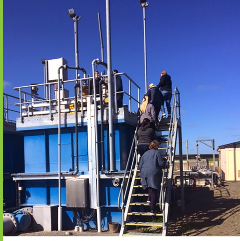
Inspecting the Palmerston North Wastewater Treatment Plant.
